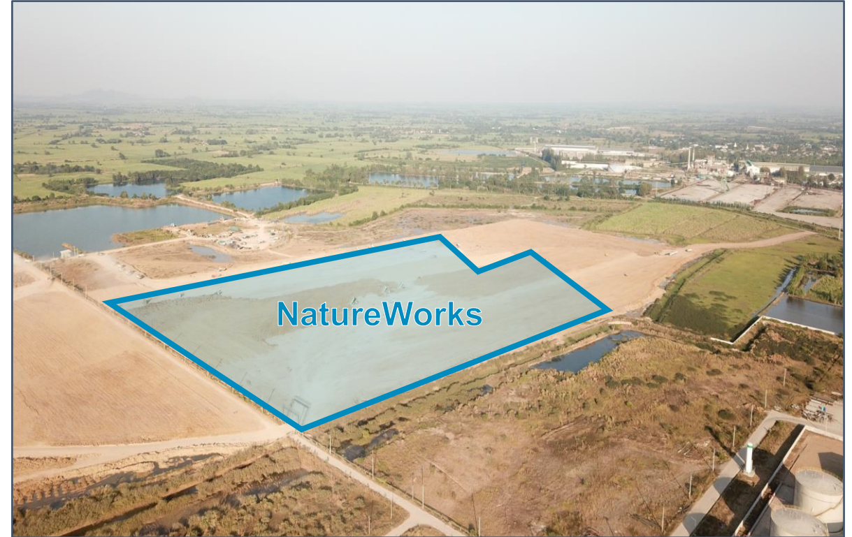
Pre-construction site of the new Ingeo PLA manufacturing facility
